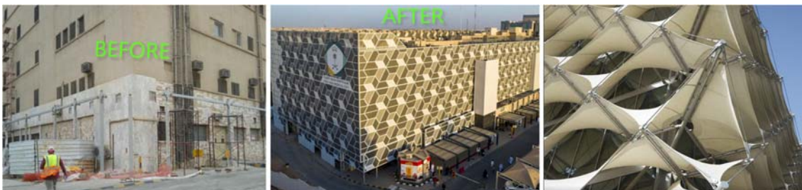
Figures 93 and 94: King Saud Medical City, Riyadh - Figure 95: King Fahd National Library, Riyadh
