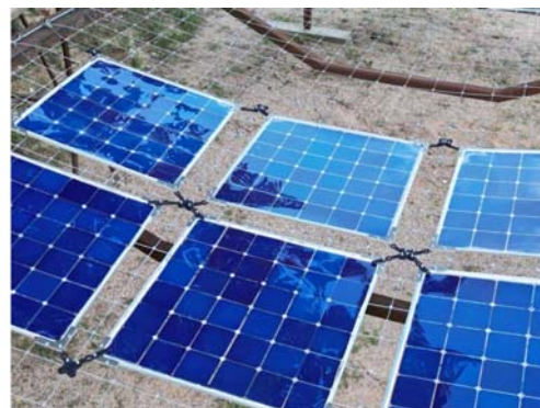
Figures 18 and 19: lightweight cable structure covered with PV modules.
