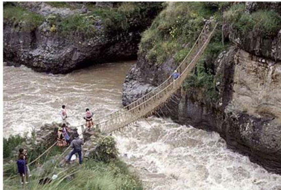
Figure 4: Rope suspension bridge under tension.
