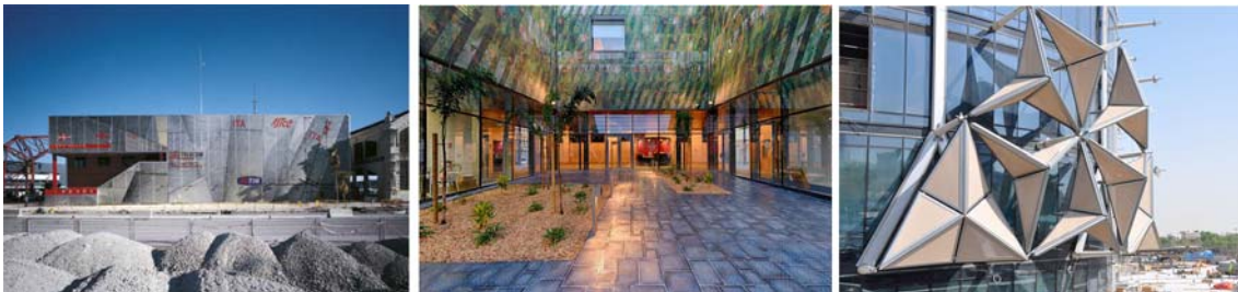
Figure 96: Luna Rossa America's Cup Base, Valencia - Figure 97: "Cours d'Appel", Fort de France - Figure 98: Al Bahar Towers, Abu Dhabi
