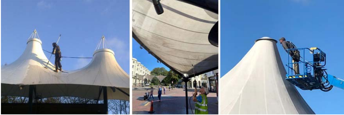
Figures 104 to 106: Maintenance and inspection.
