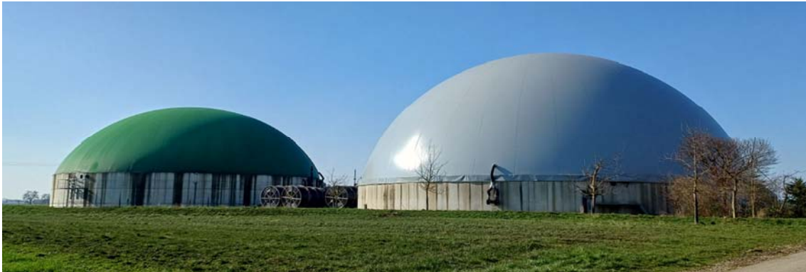
Figure 78: Biogas storage with membranes.
