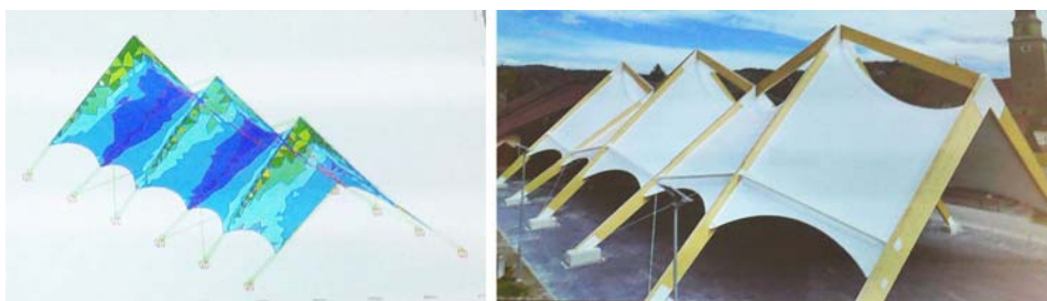
Figures 50 and 51: tent-like structure
