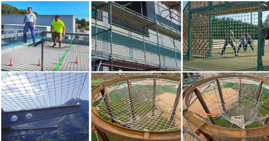
Figure 99: Work platform net - Figure 100: Side protection (railing net) - Figure 101: wire rope net for enclosure and protection - Figure 102: Horizontal net for fall protection - Figures 103 and 104: 685 kg rock fall test on Ø 6 mm wire rope net, mesh size 100 mm and specially produced steel frame
