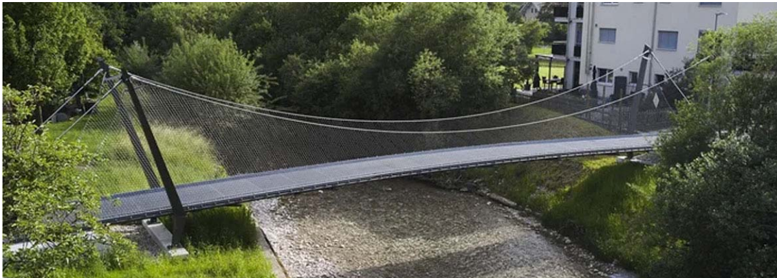
Figure 83: Himmelhausmattesteg slow traffic suspension bridge, Trubschachen, 2020
