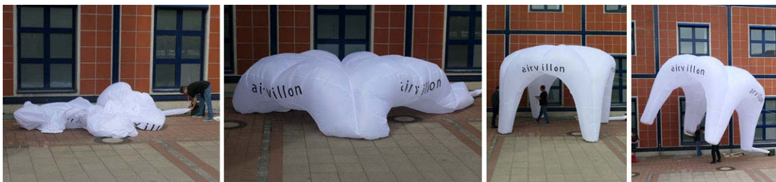
Figure 92: Airvillon, the pavilion that builds itself.
