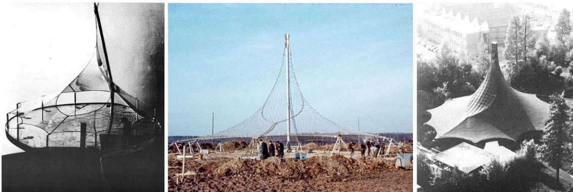
Figures 5,6: IL, Stuttgart, 1967: soap film model, cable net and as built.
