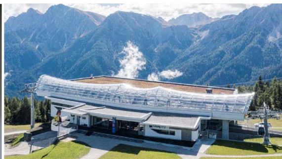
Figure 71: New Olang cable car station
