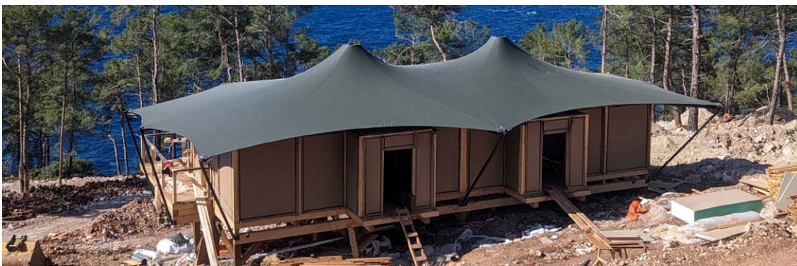
Figure 64: Almost completed project
