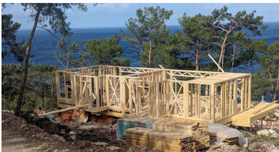
Figure 59: Wood structure for the enclosure
