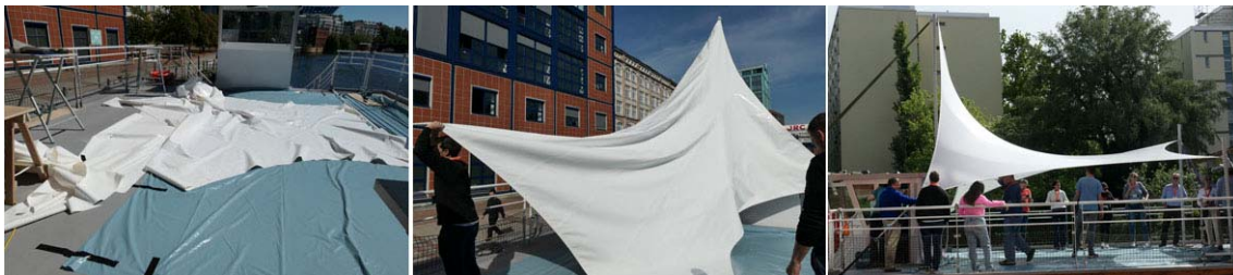
Figure 91: installation of the practical project.
