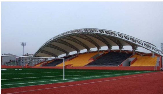
Figure 81: Firüzköy Stadium, Istanbul.
