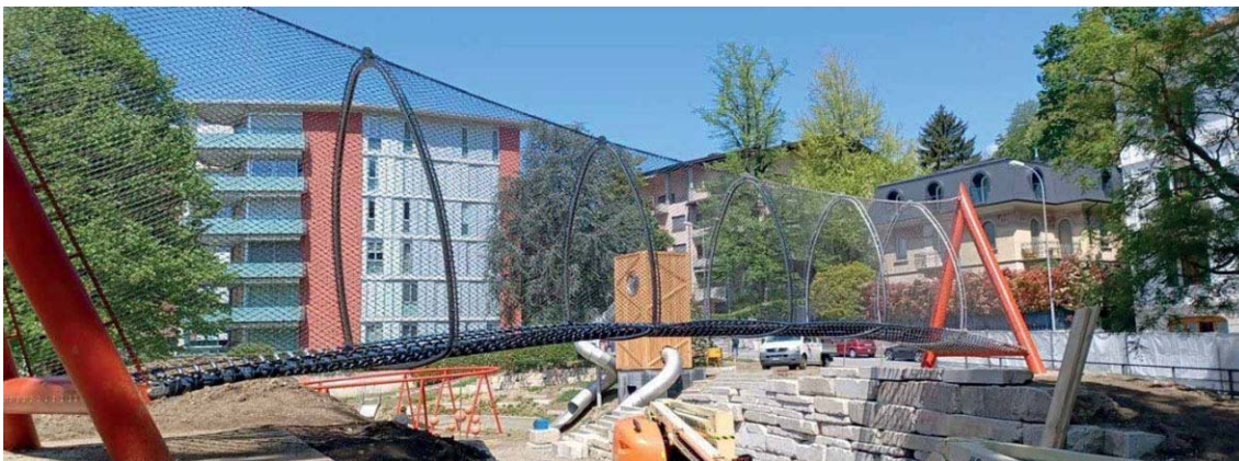
Figure 84: Webnet bridge in Lugano - Parco via Pico, 2022. Span: 15 m.
