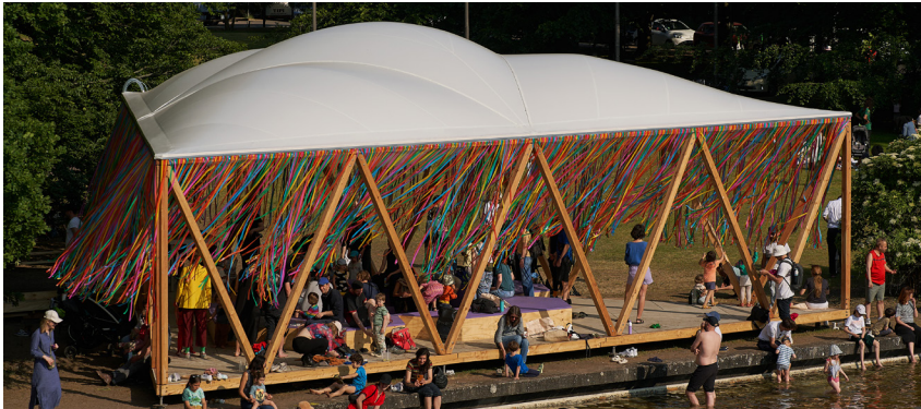
Planning, manufacturing, and installation of the roof membrane
