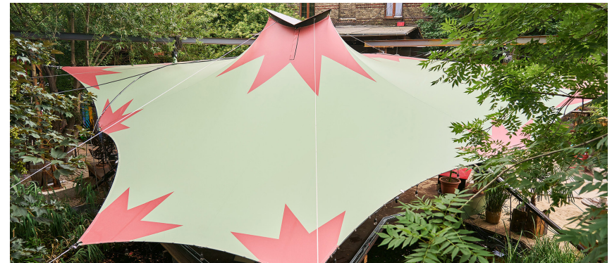
Concept, design, planning, manufacturing, and installation of the entire structure
