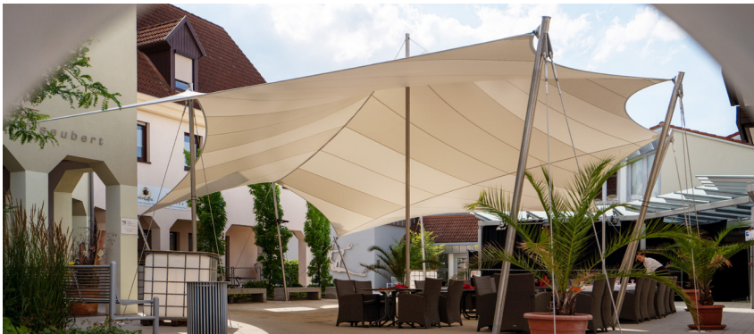
Concept, design, planning, manufacturing, and installation of the entire structure
