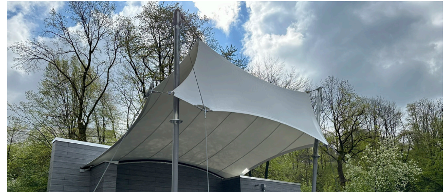
Planning, manufacturing, and installation of the entire structure
