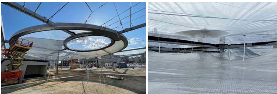
Fig.59: Installation. Fig.60: Rain during installation.
