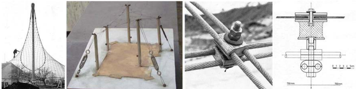
Fig.34: the "eye-loop" was invented to avoid force concentration in the net. Fig.35: small wire model. Fig.36: one of the 137.000 cable net intersection points. Fig.37: panel joint and net supporting point.
