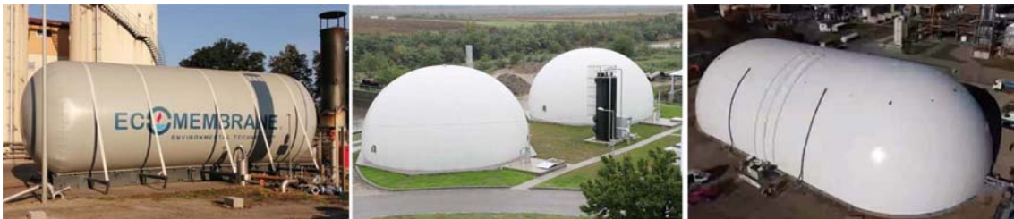
Fig. 137: gas holder on platform. Fig. 138: giant gasholders. Fig. 139: cylindrical gas holder.
