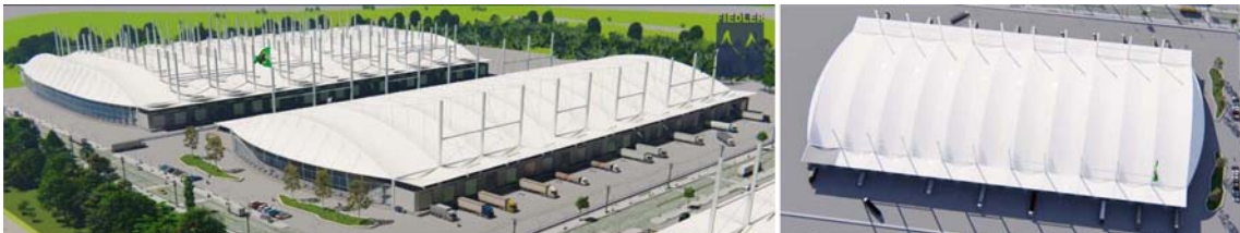
Figs.67,68: Wide span mega halls: life span over 40 years, low maintenance, lighter and cheaper than conventional halls, with natural day lighting.
