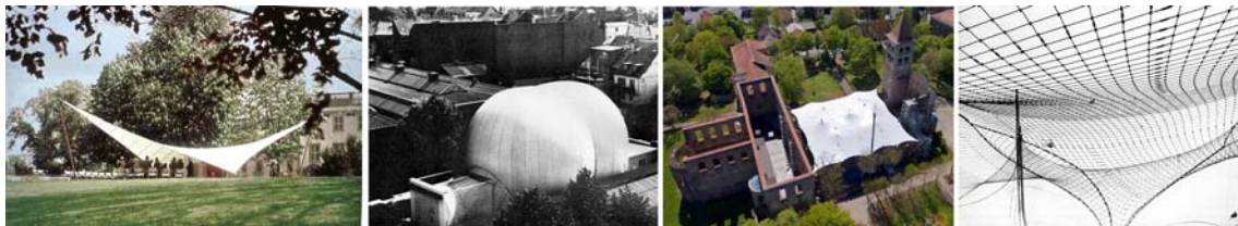
Fig.01: Music Pavilion, Kassel 1955. Fig.02: High Tension Test Station, Köln 1962. Fig.03: Convertible roof of the open air theatre in Bad Hersfeld 1968 (replaced in 2019). Fig.04: German Pavilion Expo Montreal 1967. "They arose the credo of textile buildings in Germany".
