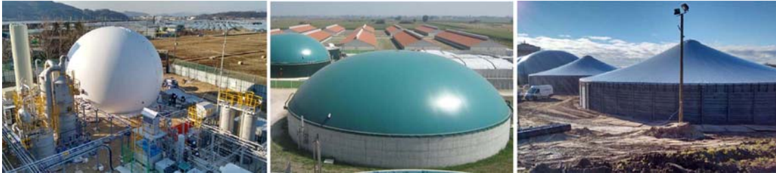
Fig. 134: gas holder on ground. Fig. 135: gas holder on tank. Fig. 136: cones.
