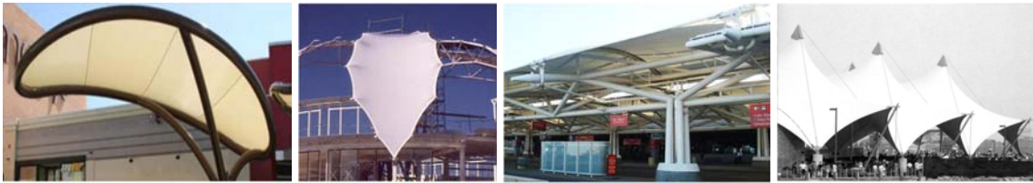
Different approaches to design the edges and the primary structure of membrane structures.
