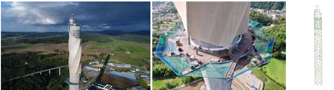
Rottweil Tower: laserscan of the concrete column.
