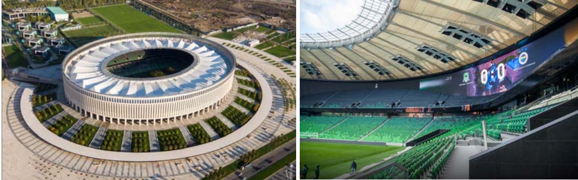
The Krasnodar Arena for 34.000 spectators is equipped with heating.
