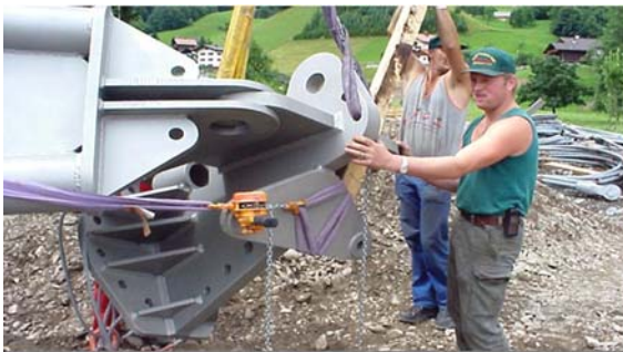
Attachment of holding devices and tensioning equipment (Courtesy of R.Off).
