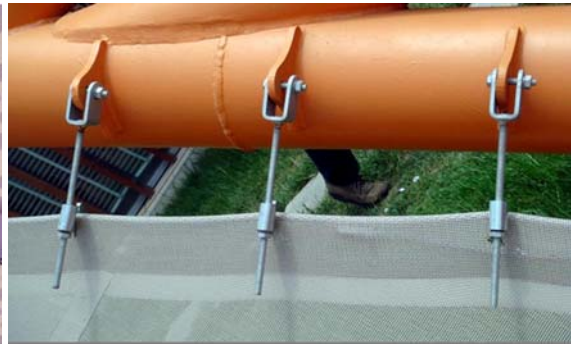
Adjustable edge for pre-tensioning through threaded rods
