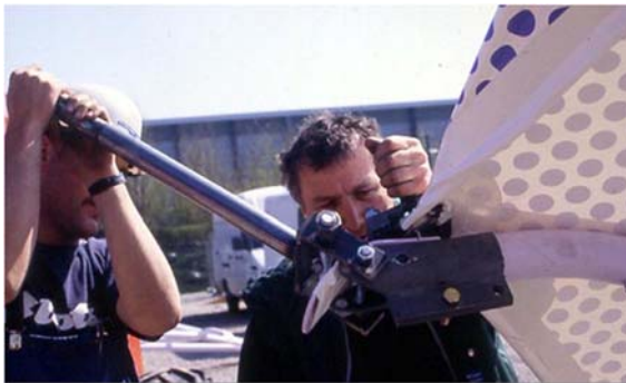
Pre-tensioning through points (A.Arnegger)
