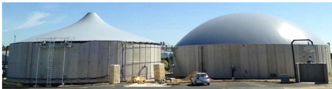
Mechanically tensioned structure(left), pneumatically tensioned structure (right)
