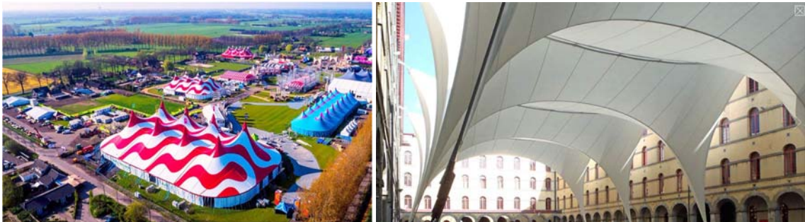
Left: 60 m yent "Texas" with separated patterns for different colours and reinforced with belts. There are not queen poles. Right: Courtyard of the "Carré des Arts", Mons.
