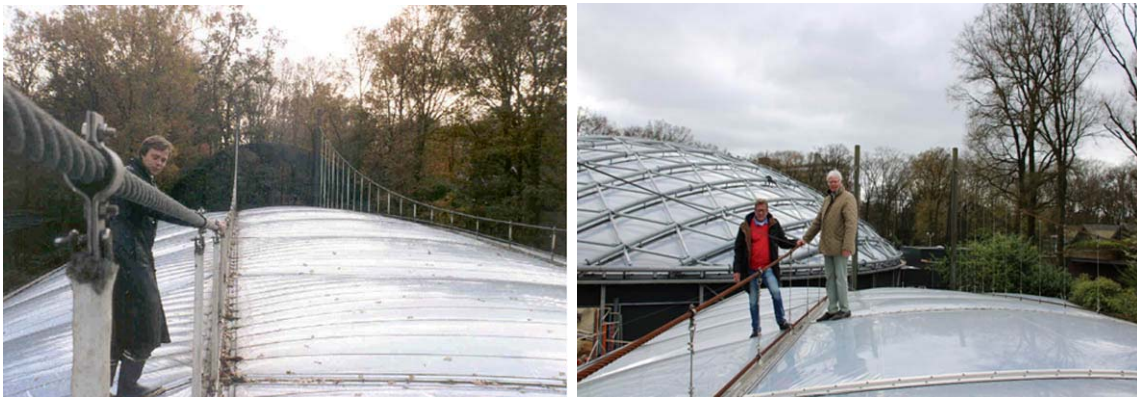
Stability of ETFE was the main topic and conclusion of Carl Maywald's lecture. First application was the 1982 Burger's Zoo in Arnhem (left) enlarged by the Mangrove Hall 35 years later (right).
