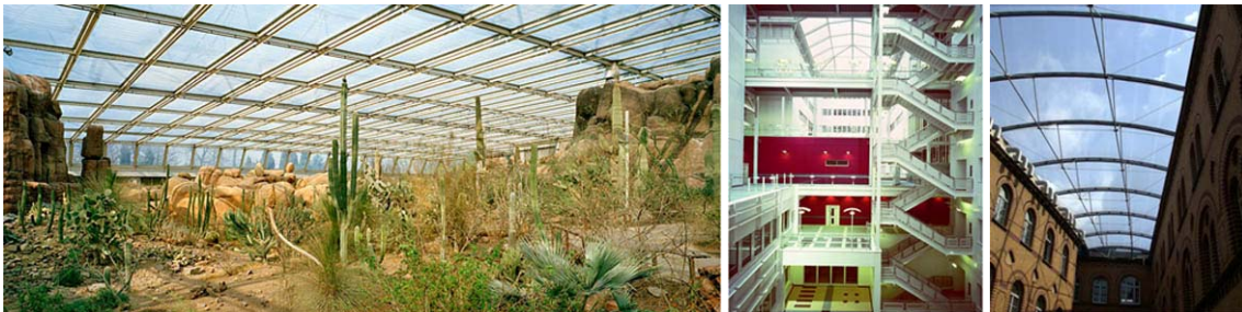
Left: Desert Hall (Burger's Zoo, Arnhem 1982). The size of the cushions was limited because of road transportation limitations. Middle: Chelsea Hospital. (London 1990). ETFE was adopted because it was cheaper than glass. Right: Aachen Kapuzinergraben 2002. The historic façade has been protected without need of columns and saving steel compared to the glazed solution.
