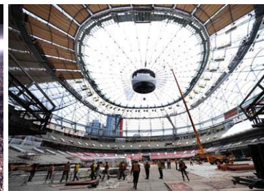
BC Place roof replacement
