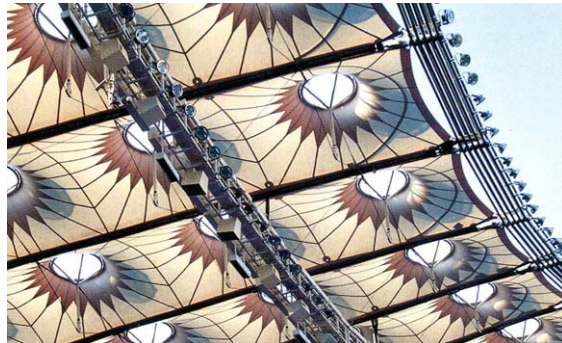
The Kiev Olympic Stadium is a single layered composition of conical shapes.
