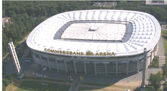
Mixed textile/polycarbonate, fixed/retractable roof of the Frankfurt Commerzbank Arena.
