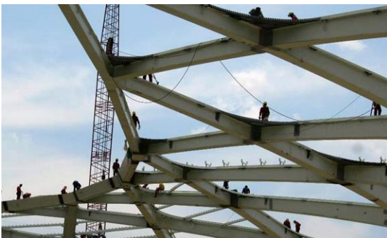
Arena de Amazonia, Manaus, with its inner compression ring.
