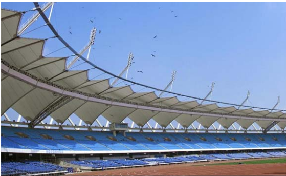
The additional roof of the Jawaharlal Nehru Stadium in New Delhi.
