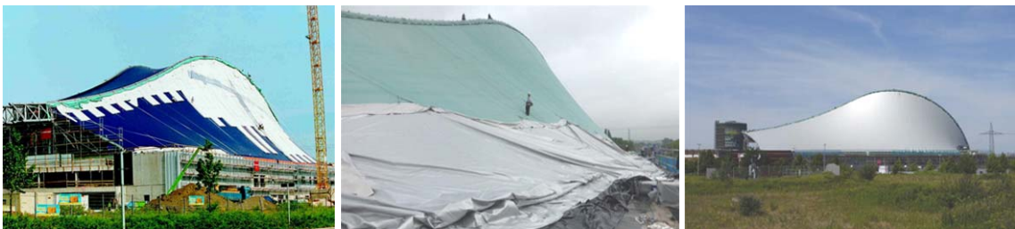
Metronom Theater, Oberhausen. PES/PVC fabric. The replacement of the outer skin while the theater was in full service.
