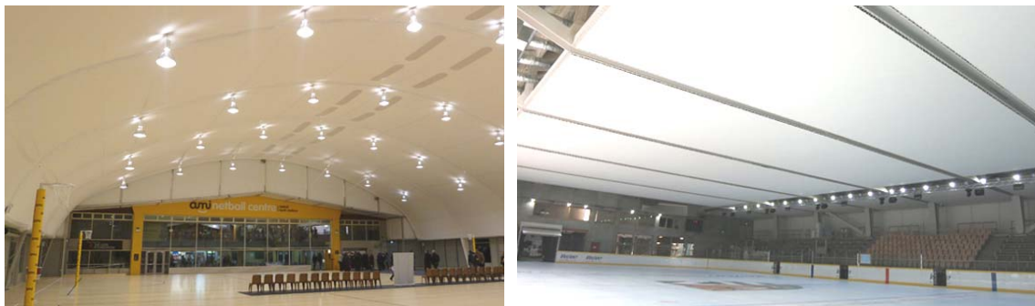
Left: in the Netball centre, Auckland, the reverberation time has been reduced from 6,95 s to 2,5 s and in the Vaujany ice skating ring (right) the reverberation time has been reduced from 7,7 s to 1,8 s.
