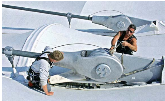
The Warsaw Stadium is notable (left) for being built above a volcano shape, its compression ring and the cables penetrating the membrane (right).
