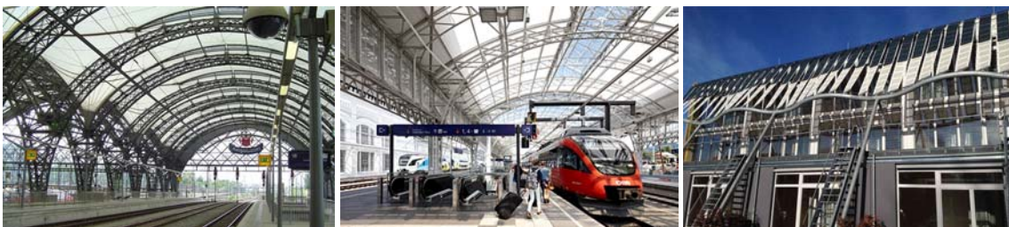
Translucency: fabric building skins and façades, which achieve visibility, protection, and energy collection.
