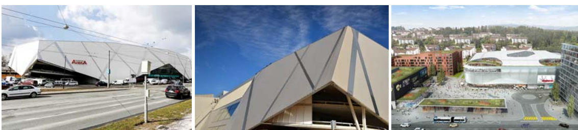
Under construction: fabric building skins and façades for protection and visibility.
