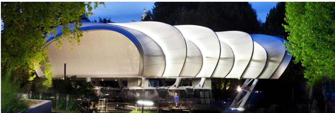
Roofing: Federal Garden Show, Koblenz
