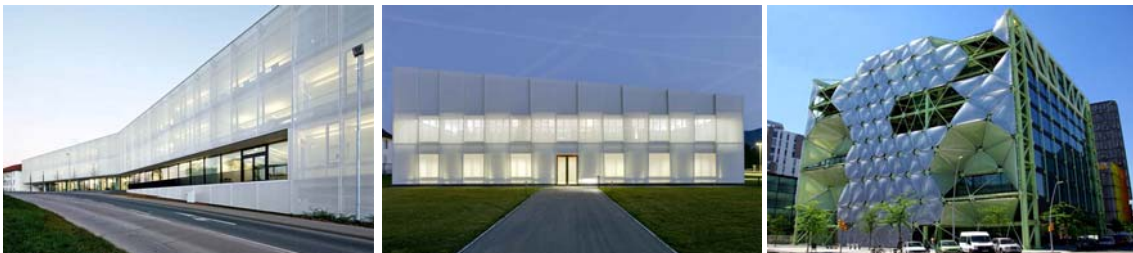
Transparent or not transparent: mesh fabrics and foil façades for shading and energy
