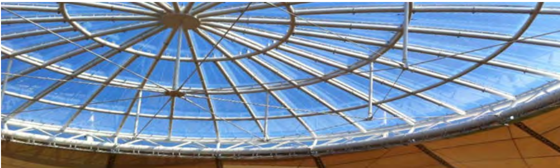
Sun Island membrane structure, Heliongjiang, 2012 (single layer)
