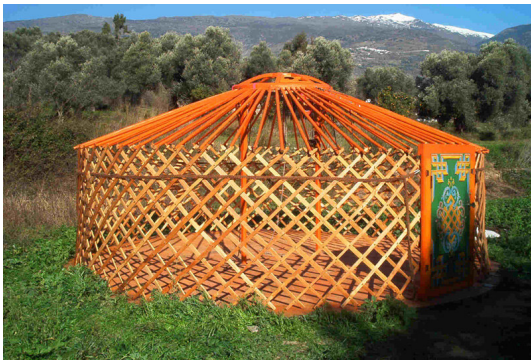
Mongolian yurt: straight lines, top ring, and vertical enclosure for transport purposes
