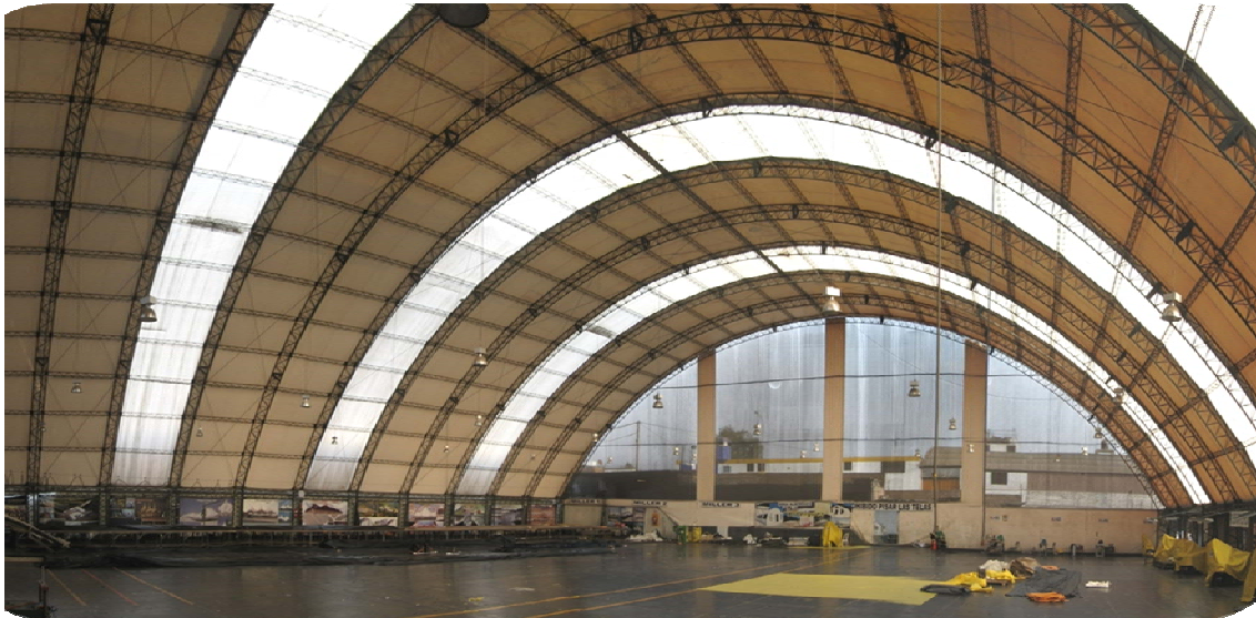
Cidelsa factory: 4.000 m 2 of steel structure + fabric
