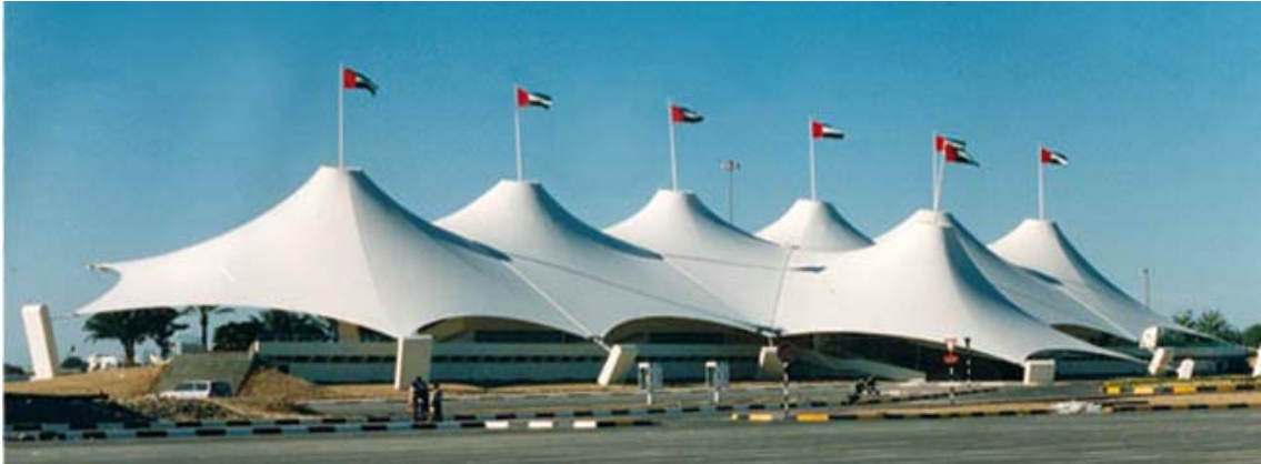
Abu Dhabi Ladies Pavillion: residual strength after 10 years of exposure: warp 89% and weft 98%
