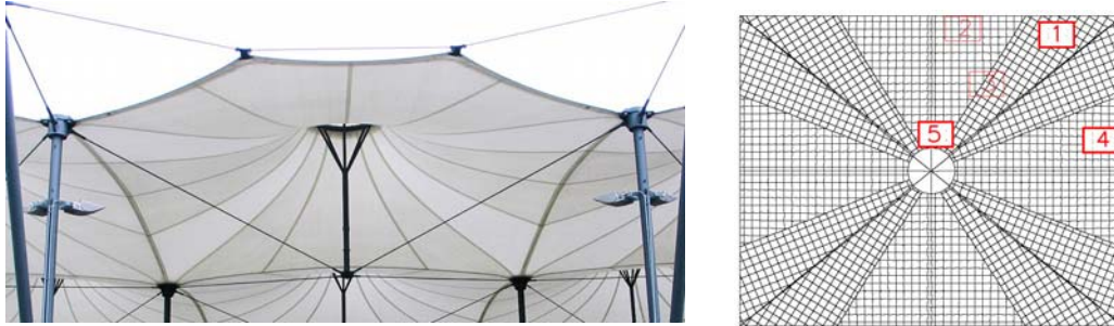
Cutting patterning of the protected parking facilities, Office for Waste Management, Munich
