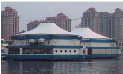
Large size membrane structures TSS-Singapore, www.tensinet.com
