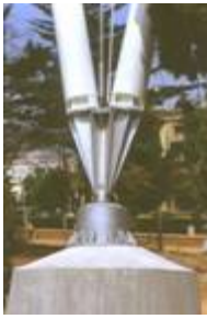
Hinged base prevents the transmission of bending
