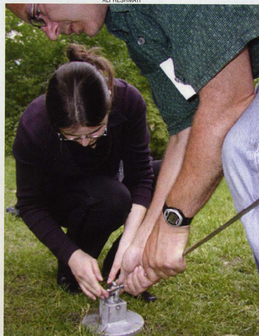
Attendees helped anchor a stay for the conference tensile structure.
