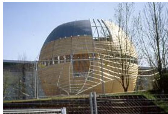
Prestressed cable net stabilizing the sphere
