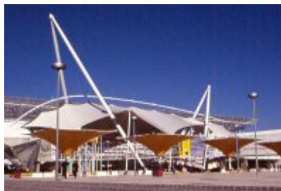
Entrance Roof, Lisbon Trade Fair. Textile as part of an integrated system
