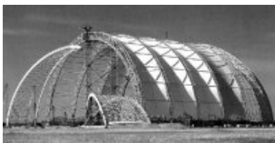
Cargo Hangar. The textile not forming part of an integrated system
