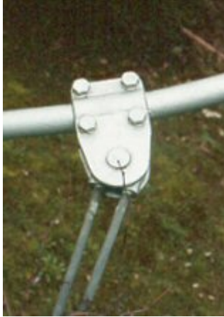
The distance between the hinge and the clamp bends the cable
