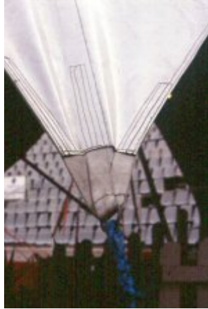
The corner does not have sufficient width and stiffness
